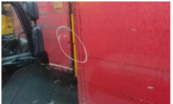
4: Bonnet Scratched Over 25mm Thru Paint
