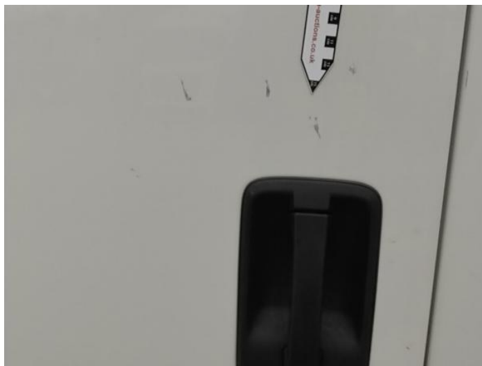
2: Door nsf Scratched Over 25mm Thru Paint
