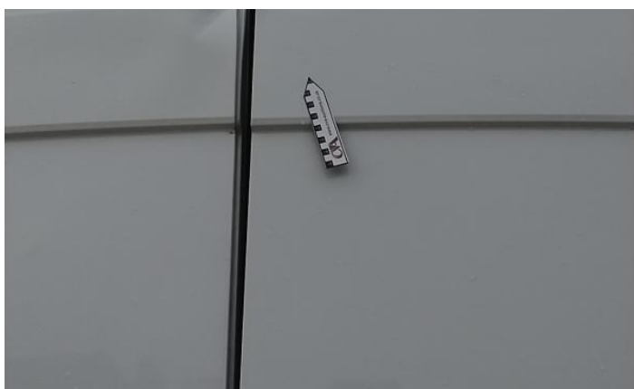
11: Door nsr Dented Over 30mm
