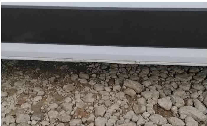
5: Door nsr Scratched Over 25mm Not Thru Paint
