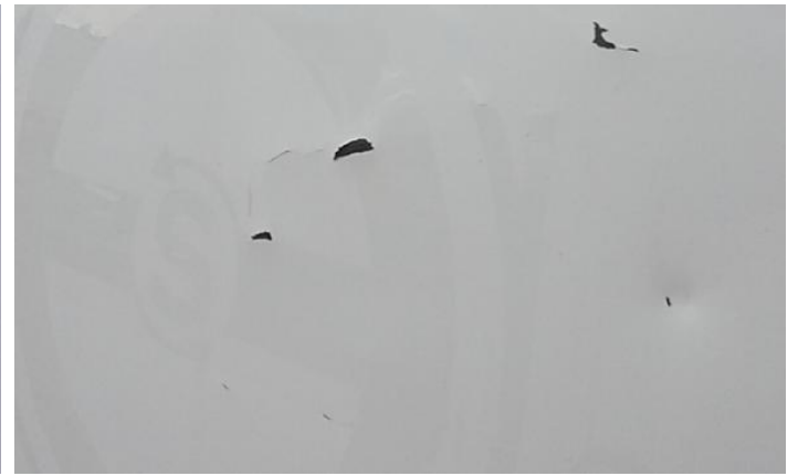
10: Door osr Chipped Multiple Chips
