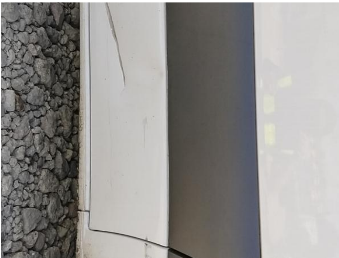
23: Door osf Dented With Paint Damage
