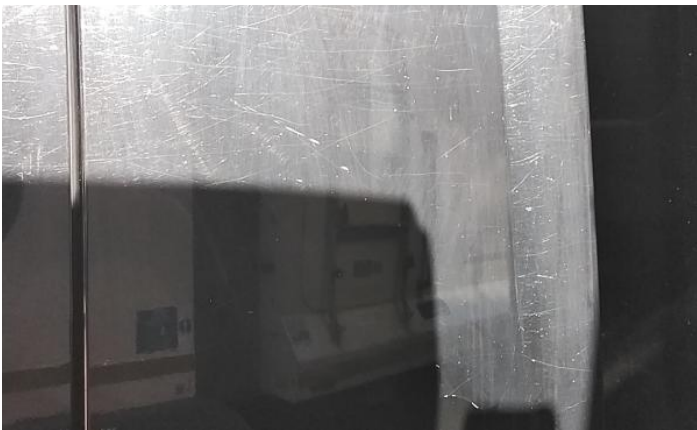
5: Door nsf Scratched Over 25mm Thru Paint
