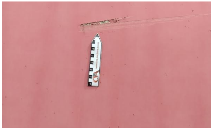
6: Door nsf Chipped Multiple Chips
