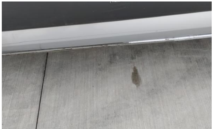
12: Sill ns Dented With Paint Damage
