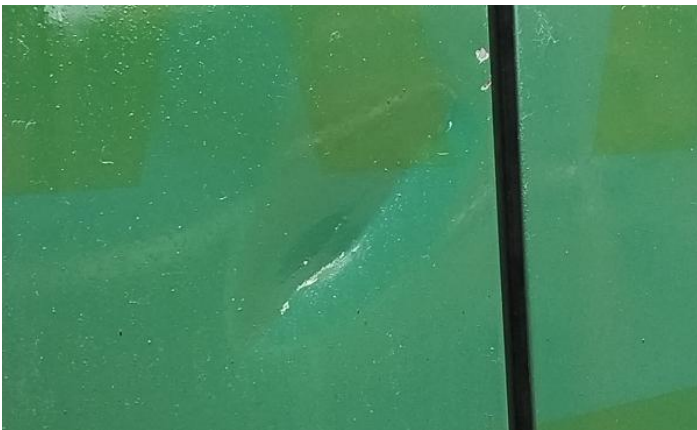
5: Panel Rear Chipped Over 5mm
