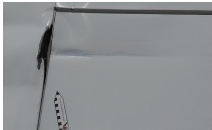
15: Door osr Dented With Paint Damage
