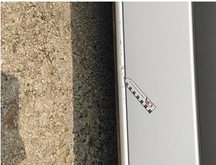
5: Sill ns Dented With Paint Damage
