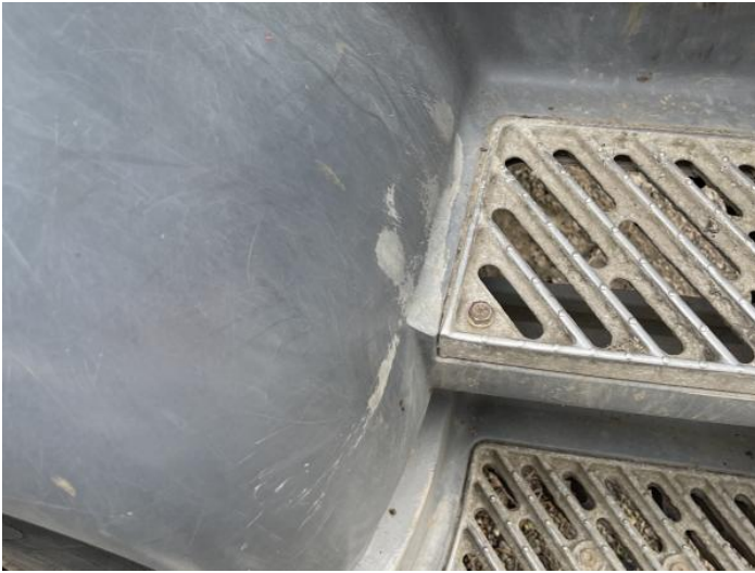
3: Door Moulding osf Scuffed (Unpainted) Over 100mm
