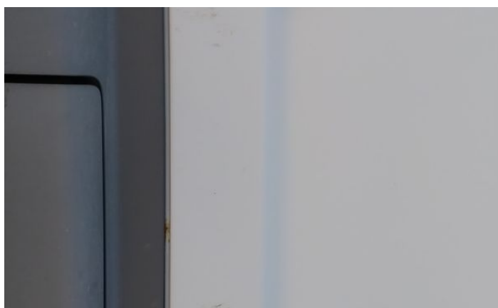
6: Door nsf Scratched Over 25mm Thru Paint
