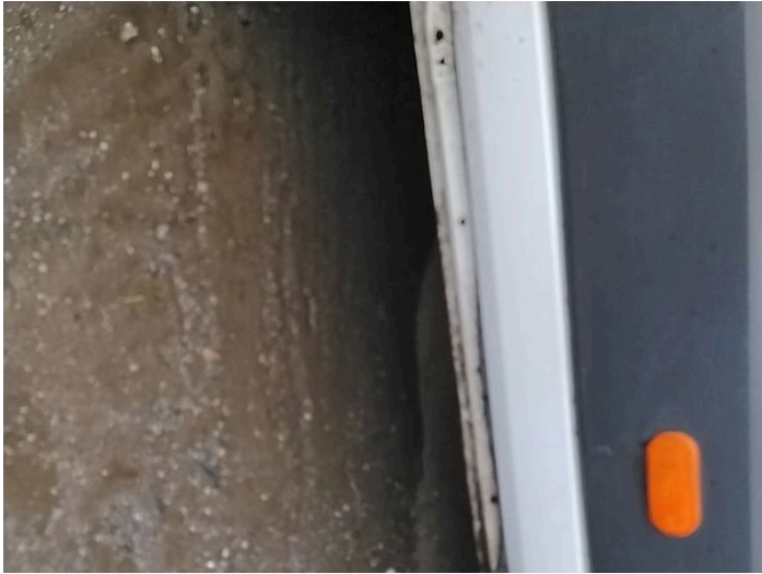
6: Door Moulding nsf Missing Replace
