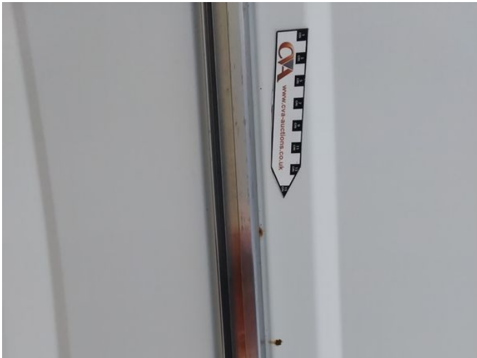
13: Qtr Panel nsr Rusted Over 5mm
