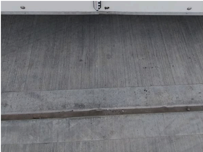
7: Sill os Dented Over 30mm
