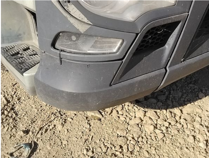
1: Bumper Front Moulding Broken Replace
