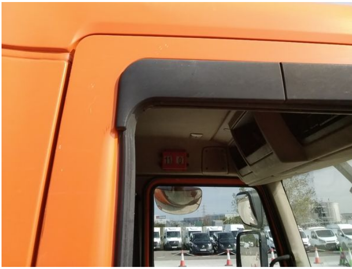
33: Roof Dented Over 30mm
