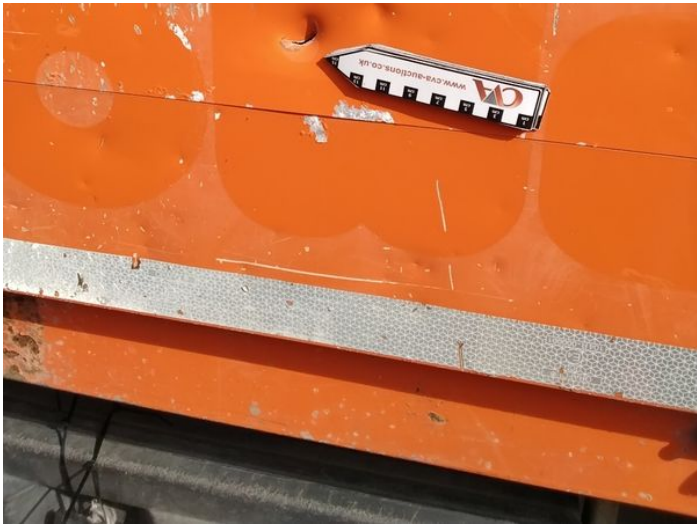
25: Qtr Panel osr Hole Over 10mm
