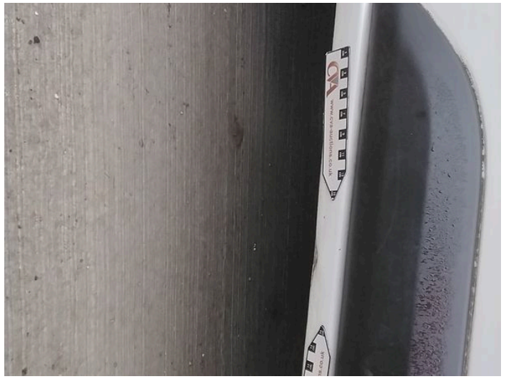
10: Sill os Dented With Paint Damage
