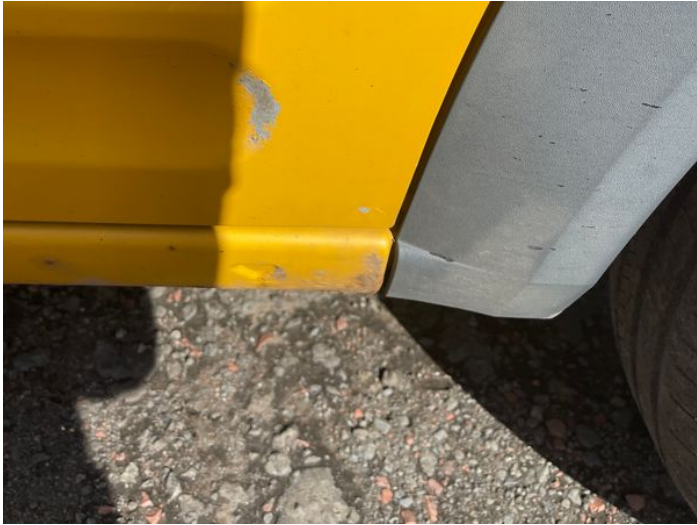
6: Door nsr Rusted Over 5mm
