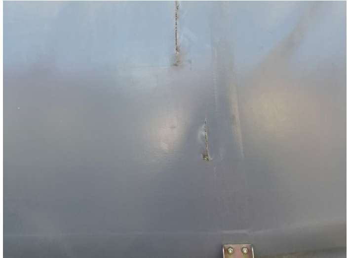
2: Qtr Panel nsr Hole Over 10mm
