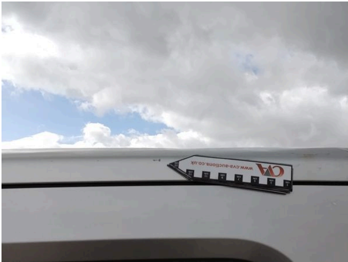
8: Roof Chipped Over 5mm
