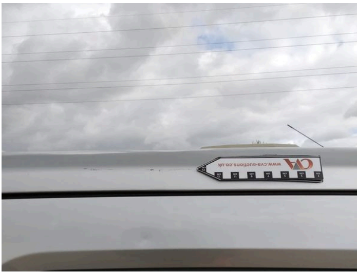
9: Roof Chipped Over 5mm
