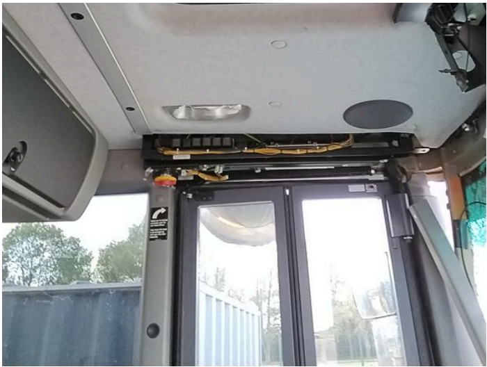
21: Switches And Controls Missing Replace
