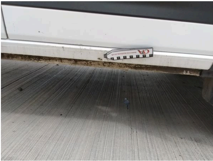
10: Sill os Chipped Over 5mm
