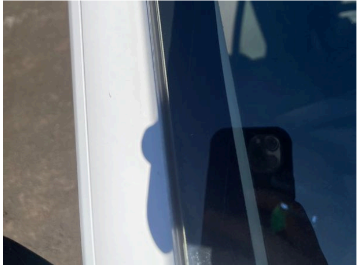
2: Panel Front Scratched Over 25mm Thru Paint
