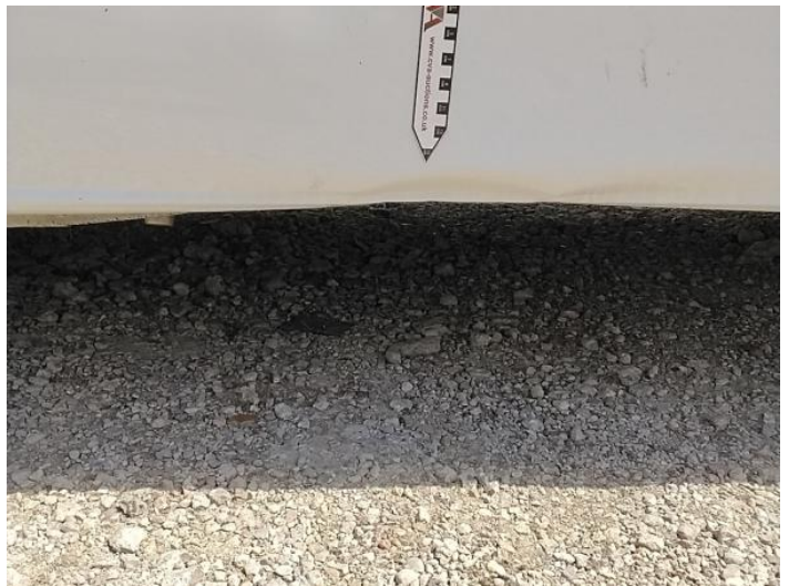
6: Sill os Dented Over 30mm
