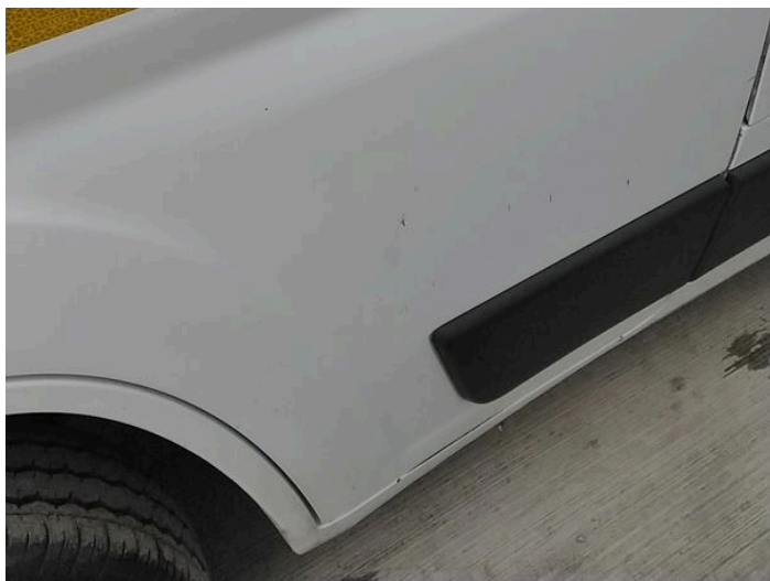
5: Door nsf Chipped Multiple Chips
