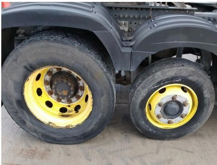
10: Wheel osr Corroded Light
