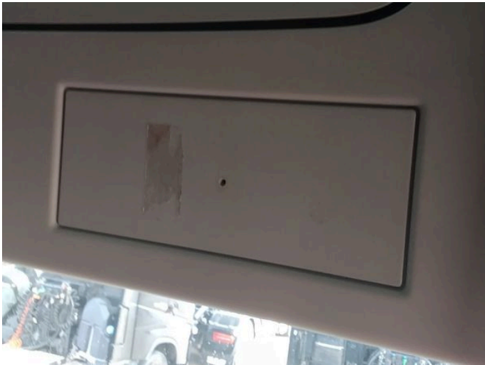
25: Centre Console Front Holed Over 3mm
