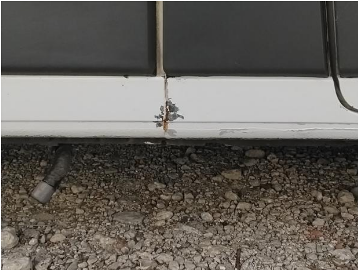
9: Sill os Rusted Over 5mm
