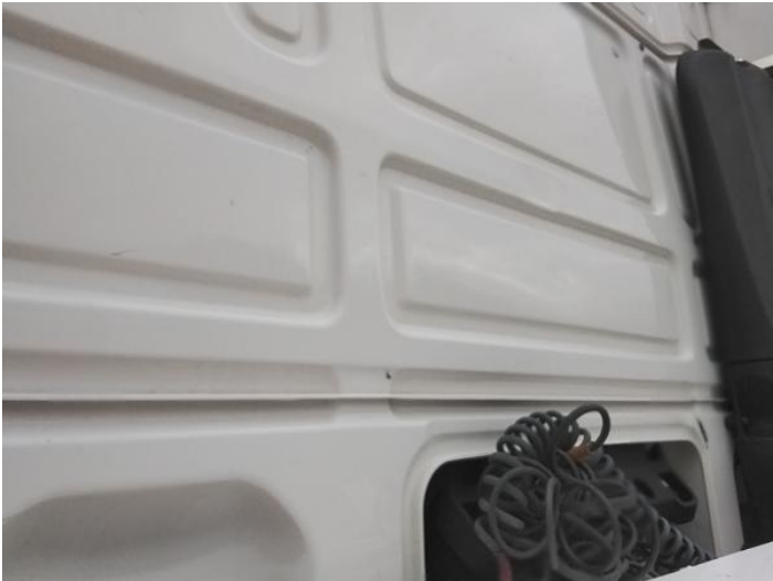
3: Panel Rear Dented Over 30mm
