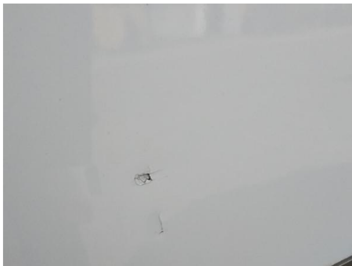
4: Door nsr Hole UpTo 10mm
