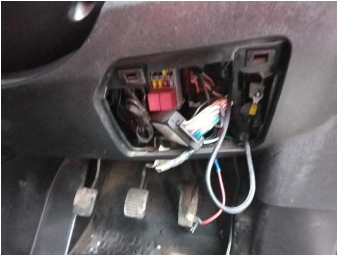
15: Fascia Panel Missing Replace
