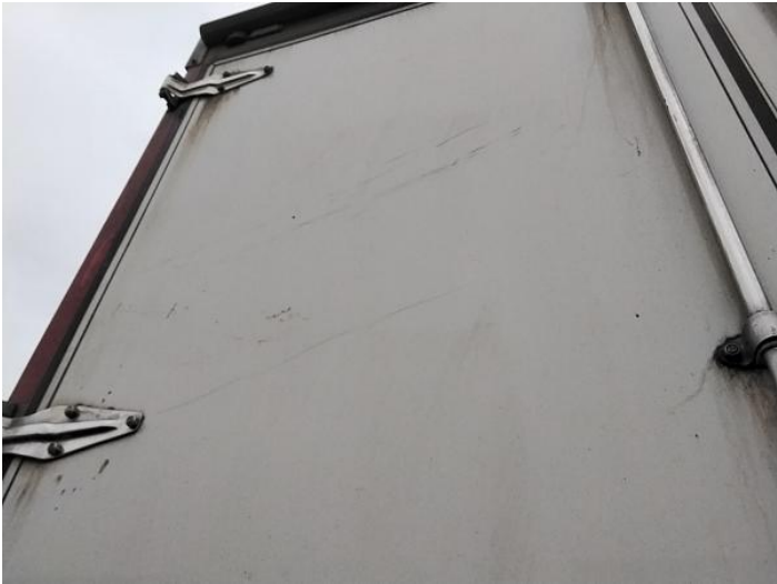
9: Door nsr Scratched Over 25mm Thru Paint
