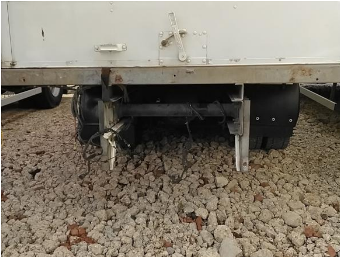
9: Number Plate Rear Missing Replace
