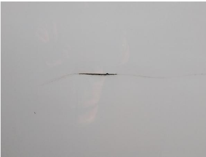
5: Qtr Panel nsr Cracked Replace
