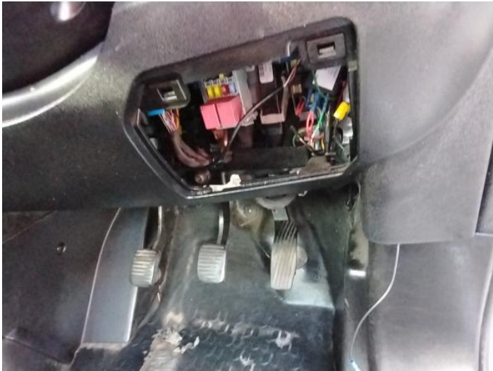
10: Fascia Panel Missing Replace
