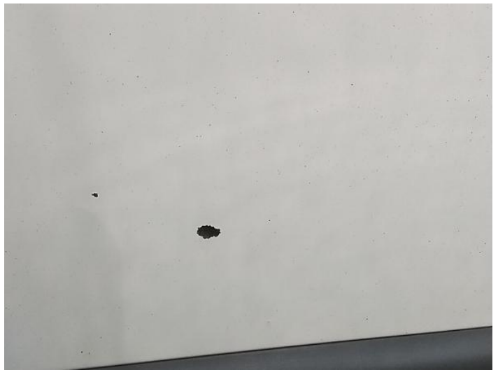
6: Panel Front Chipped Over 5mm
