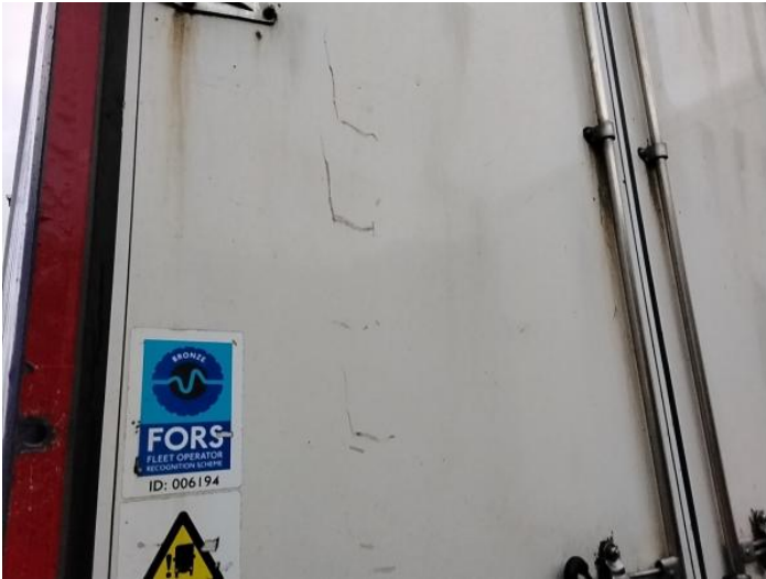
3: Door nsr Scratched Over 25mm Thru Paint
