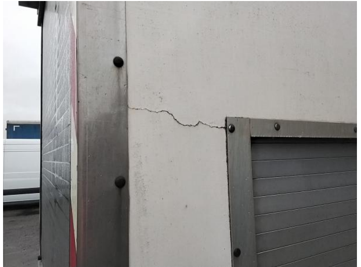
4: Qtr Panel osr Cracked Replace
