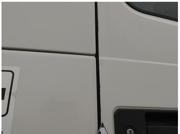
14: Door osf Chipped Edge Chip
