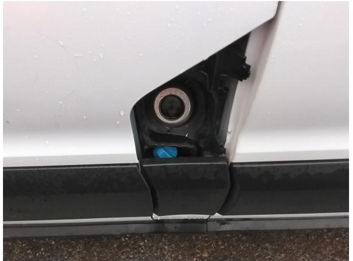
4: Fuel Flap Missing Replace
