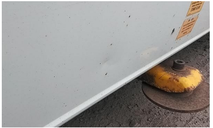
4: Panel Front Chipped Multiple Chips
