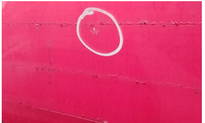
10: Door osf Scratched Over 25mm Thru Paint
